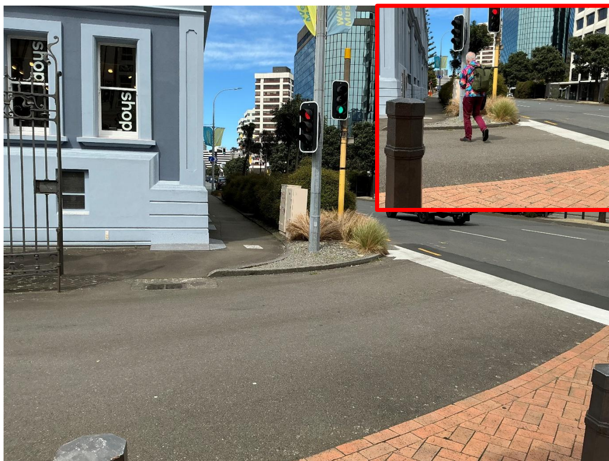
Figure 5-6: View of exit from TSB Arena. Note lack of hold line. INSET: Pedestrian desire line.
