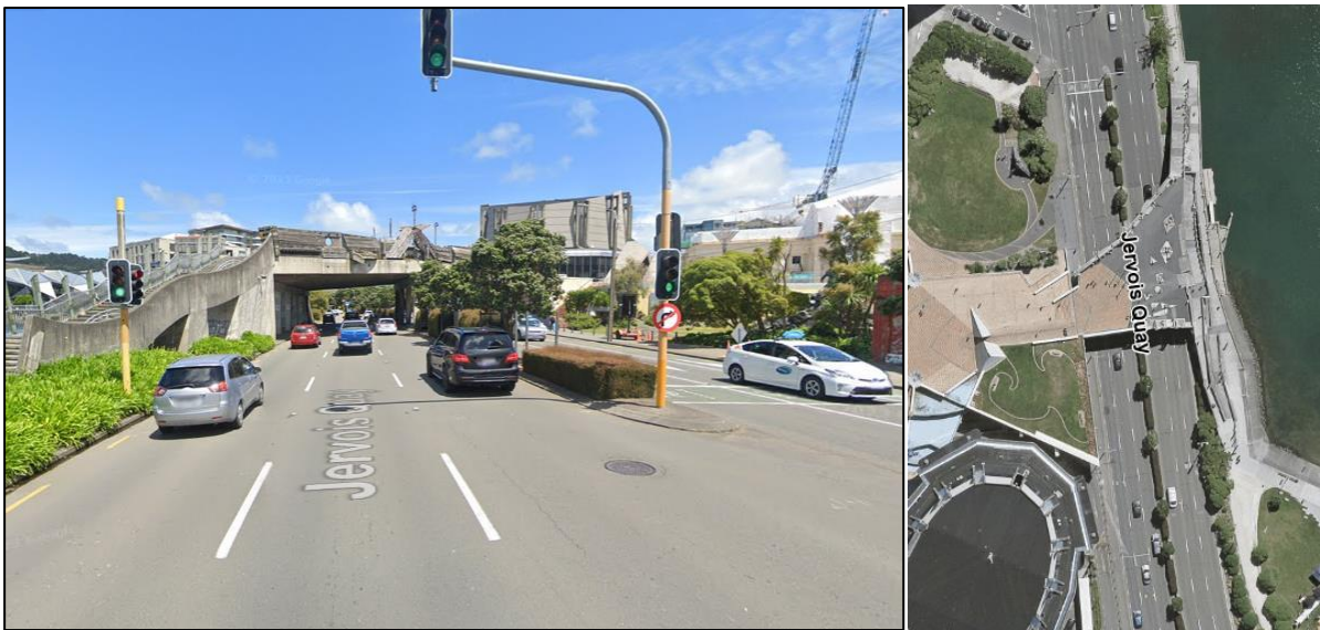
Figure 1-9: City to Sea Bridge over Jervois Quay (Source: Google Maps Streetview and WCC Wellington Maps)
