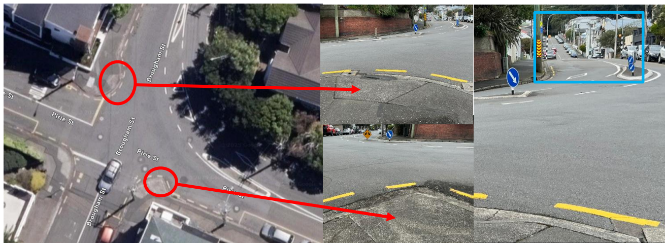
Figure 5-2: Pedestrian drop kerbs (cut downs) that should be removed.
